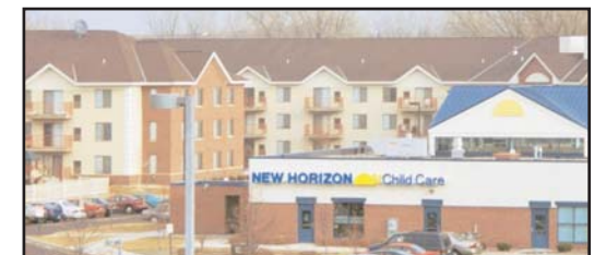
Below, the site includes the New Horizon Child Care Center and the Dakota Station Apartments.
